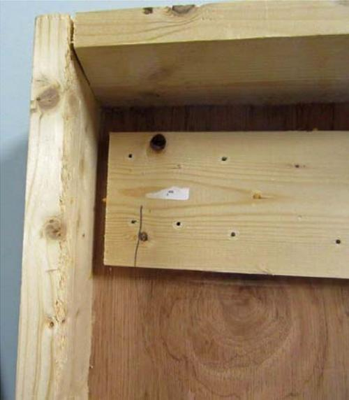
A poorly designed support for the legs is not attached to the frame.
