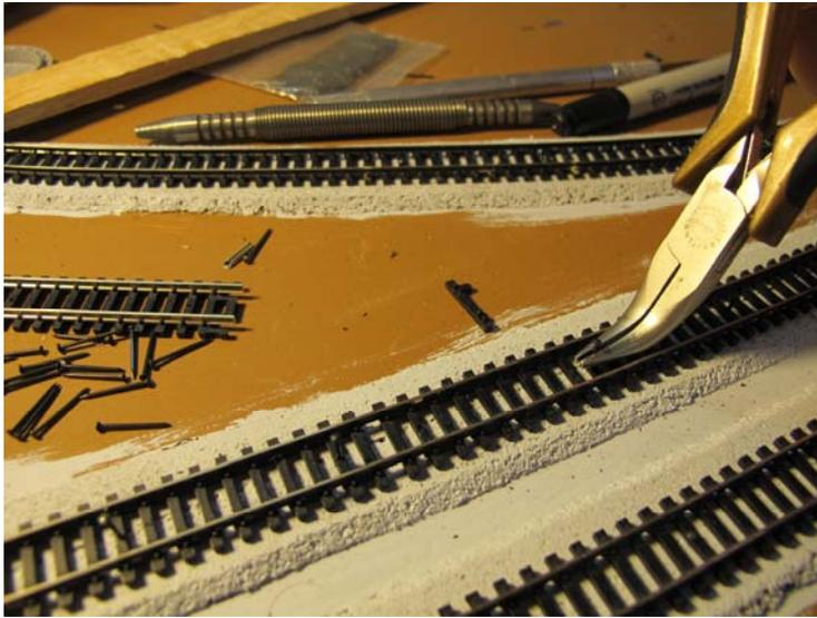
8. Make a mark on the roadbed between 5 1/4 and 5 1/2-inches at the other end of the module to leave room for a short section of straight track at that end.
